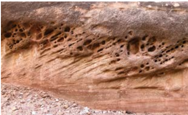
Tafoni in a cliff face made of the Navajo Sandstone. These tafoni are preferentially oriented along the cross-bedding that formed during deposition in a sand dune environment.
