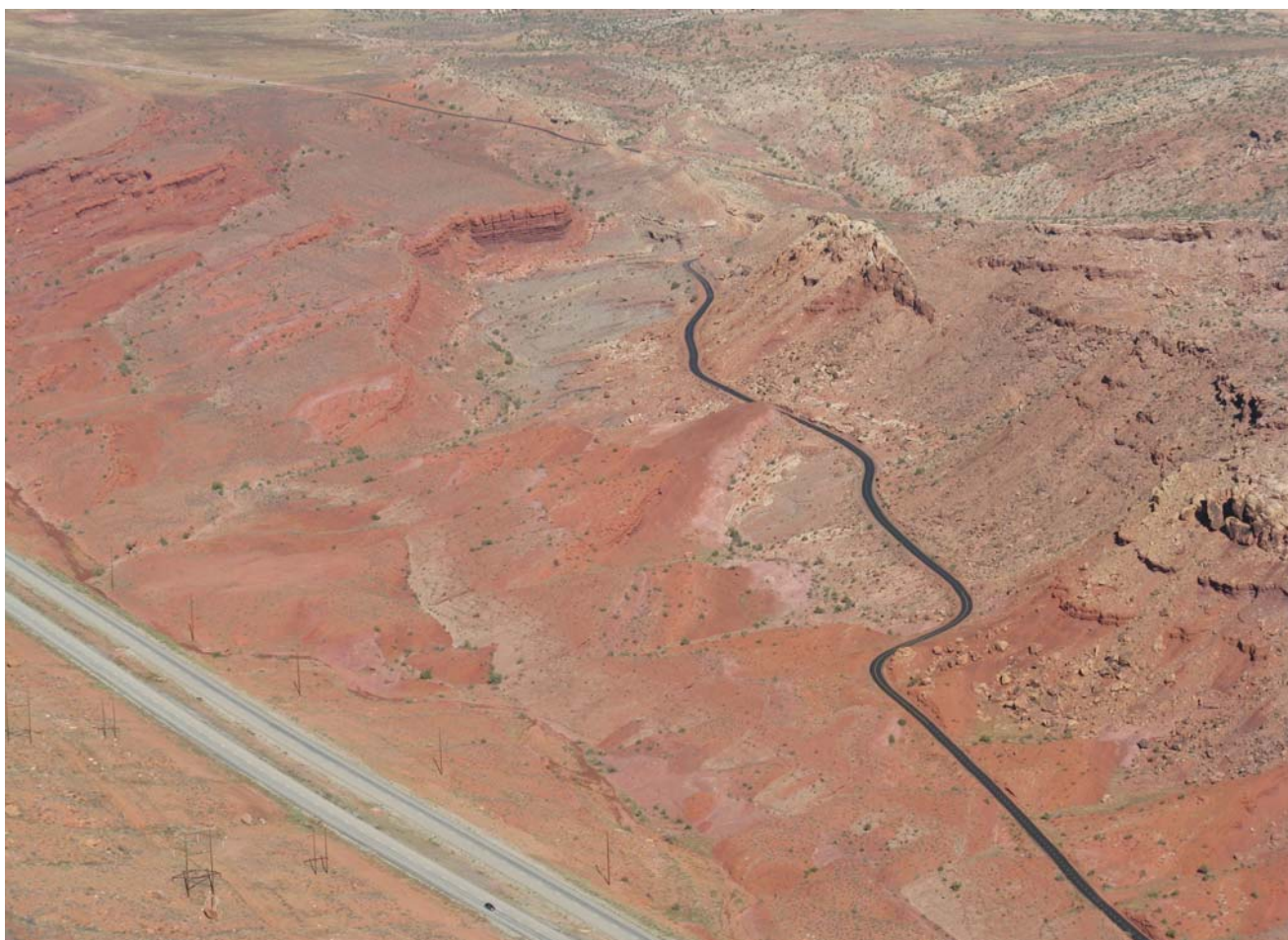
Old Highway new bike path.
