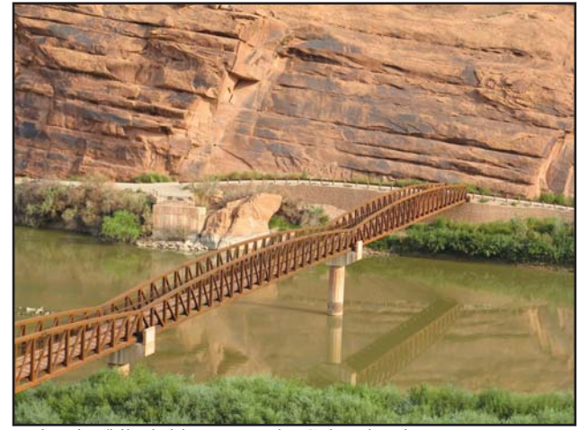
Pedestrian/bike bridge across the Colorado River
