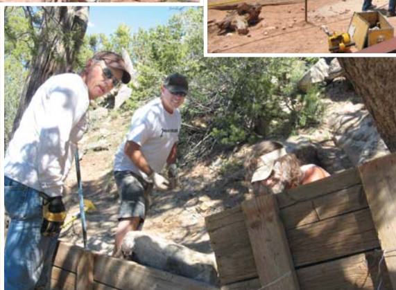
Shoring up eroded trail
