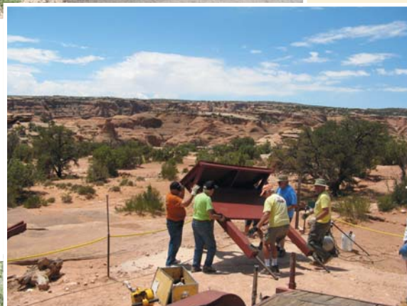
Shoring up eroded trail
