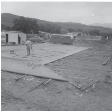
Building of the wood floor of Moab's first skating rink began the summer of 1955.
