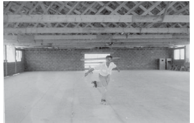
Skating rink co-developer Harold Jones roll tests strength of redwood floor as work continues on trusses above.
