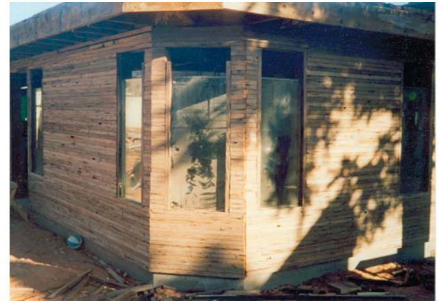
Much of John Lillibridge's house was built using 2x2-inch skating rink slats for flooring, an addition, decking and decorative exterior.
