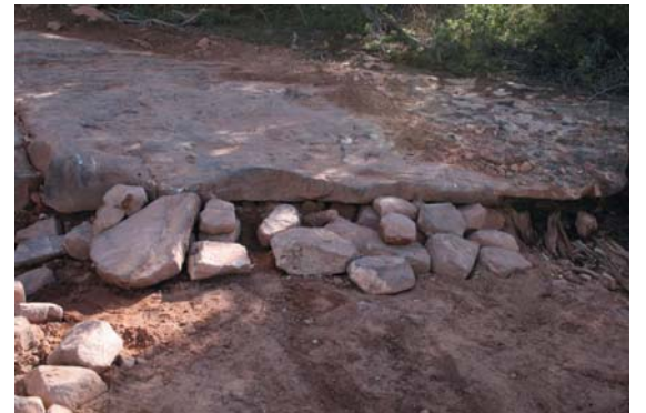
Some obstacles may require building ramps out of stones in order to continue.
